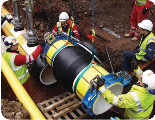
630mm bag-off and tee insertion operation
