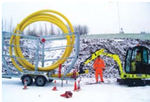
Radius gas pipe coils being used at JCB's HQ
