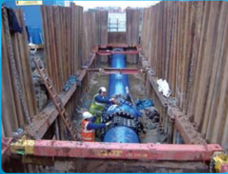
Typical excavation and assembly
