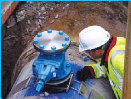
The Radius PE air valve being installed, with minimal excavation required
