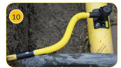
The Anaconda® connection is complete. The installation should be tested before commissioning
