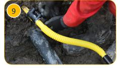
Once the fitting is fully cooled, remove all the clamps
