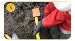
When the tapping tee is fully cooled, mark and prepare the Anaconda® pipe spigot end
