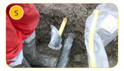
Install the fitting on the service pipe up to the pipe stop. Keep the packaging on the fitting to protect from contamination
