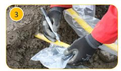
While the tapping tee is cooling, prepare the service pipe end. Mark the socket insertion depth and the area on the pipe to prepare
