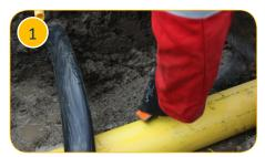
Mark the position of the fitting on the main, using an approved marker pen and prepare the pipe surface area with a pipe scraping tool
