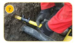
Insert the Anaconda® pipe spigot end into the fitting on the service pipe up to the pipe stops
