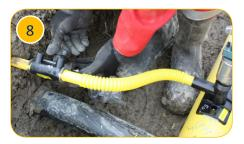
Clamp the fitting in place. Where necessary, support the joint to prevent sagging. Weld the fitting following industry best practice
