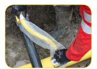
The flexible pipe minimum bend diameter = 90mm.
