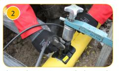
Clamp the tapping tee body on the prepared surface and weld following industry best practice
