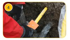
Using an approved pipe preparation tool, scrape the pipe surface
