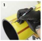
Ensure the pipes to be joined are free from damage and are cut square. Using an approved marker pen, mark a minimum of 25 mm around the pipe's circumference.
