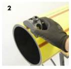
Using the ProFuse pipe exposure tool (PET™), score the external skin around the circumference of the pipe.
