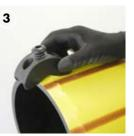
Rotate the PET<sup>™</sup> 90° and score the external skin longitudinally towards the pipe end.
