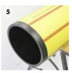
Skin removed. Repeat steps 1 to 4 for the second pipe to be joined. Follow industry best practice when making the butt-fusion joint.
