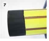
Skin removed. If the pipe surface becomes contaminated after skin removal, re-prepare the pipe using industry approved pipe surface preparation tools.
