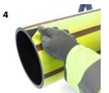
Lift the edge of the skin as shown above and peel the skin away from the core pipe.
