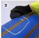
Using the ProFuse pipe exposure tool (PET<sup>TM</sup>), score the external skin around the marked area.
