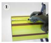
Ensure the pipes to be joined are free from damage and are cut square. Using an approved marker pen, mark the fitting's insertion depth + 25 mm.
