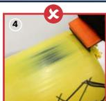
Treat the pipe as a conventional PE pipe. DO NOT remove all of the yellow outer surface as this may lead to a poor quality joint.
