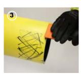
Prepare the pipe surface using an industry approved pipe surface preparation tool.
