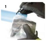
Ensure the pipes to be joined are free from damage and are cut square. Using an approved marker pen, mark the fitting's insertion depth + 25 mm.
