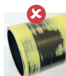
Incorrect pipe preparation for electrofusion
