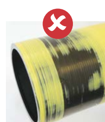
Incorrect pipe preparation for electrofusion
