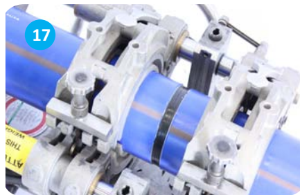
17 2. Pipe check cycle The automated jointing phase can begin
