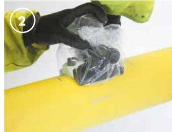
2 Using the saddle fitting as a guide, mark the outline area of the pipe to prepare for electrofusion jointing, using an approved marker pen.
