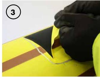
Lift and pull the edge of the outer skin away from the core pipe and peel the skin. Take care not to contaminate the pipe surface.
