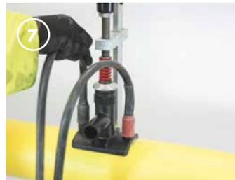
7 Connect the electrofusion control box terminal leads to the fitting and follow the instructions on the control box.
