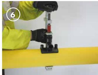
6 Using an approved calibrated clamp, secure the saddle fitting in place. Ensure the correct clamping force is applied (check clamp indicator).
