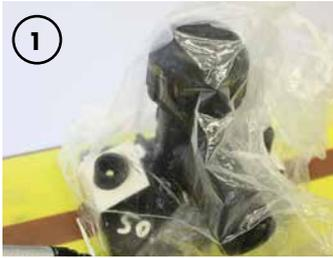
Using the tapping tee as a guide, mark the outline area of the pipe to prepare for electrofusion jointing, using an approved marker pen.
