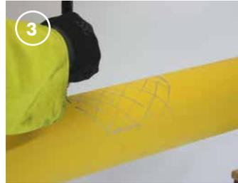
3 Mark the area as shown using a cross hatch pattern to indicate the area to be prepared.
