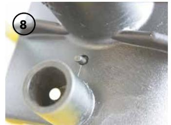
8 Melt indicators show that the fusion process has taken place. It is not confirmation of a quality joint. Clamps must remain in place during the full cooling period.
