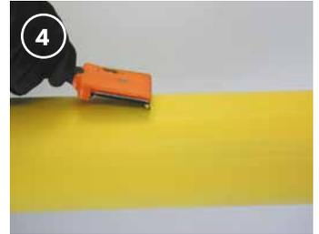
4 Prepare the pipe surface using an industry approved hand scraping tool.
