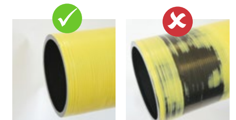
Correct pipe preparation for electrofusion
